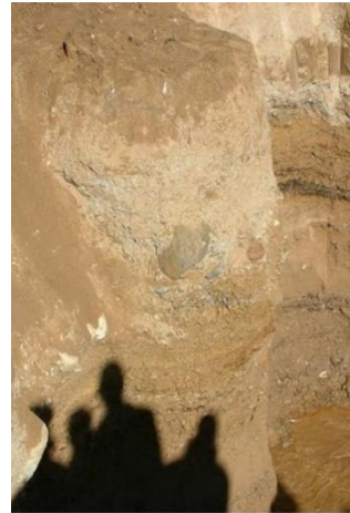
FIGURE 8. - Jet grout column [26].
