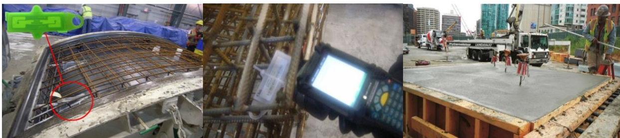
FIGURE 4. - RFID technology is being employed in the concrete structures [downloaded from Google].
