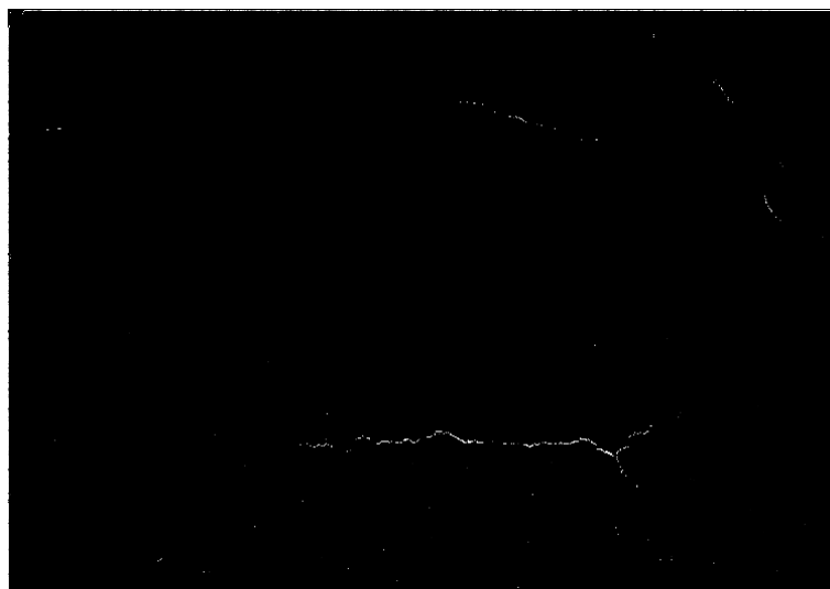
FIGURE 5 Final image after segmentation with the cracks
